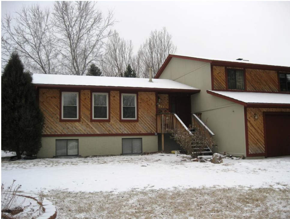
Front view of the home
